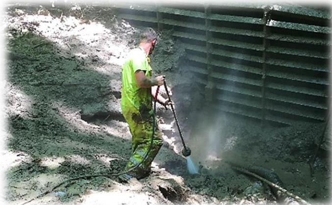
Using the power washer to create a slurry that can be vacuumed to the truck. Photo courtesy Todd Strole
