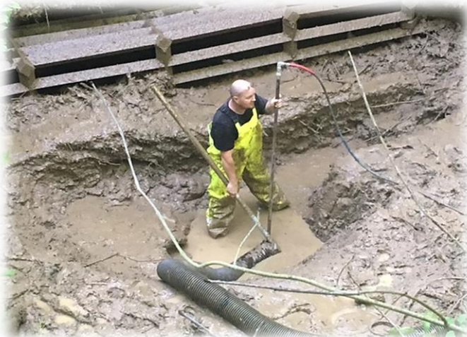
The first day of silt removal. A small "dam" of material was left along the gate as the project progressed to minimize the amount of silt and debris re-entering the cave. Photo courtesy Terry Esker
